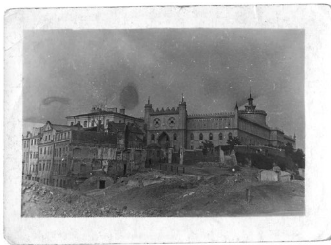
Ruins of Szeroka Street, c. 1943 (unknown photographer, Photographic Collection of Municipal Preservation Projects / Municipal Historic Preservation Office)
