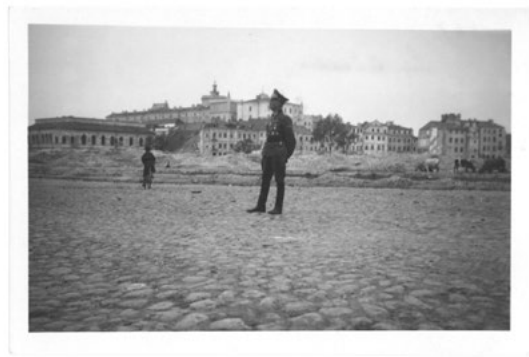
Ruins of the Jewish quarter: Maharshal Synagogue, partially dismantled; remains of Szeroka Street at the foot of Castle Hill, 1943 (unknown photographer, Marek Gromaszek collection)
